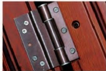
Strengthened hinges, Thicker, more flexible
