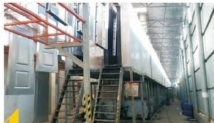
Chemical treatment for the steel sheet to make it rust proof
