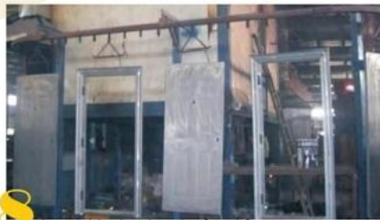
Assemble the door leaf and frame together and do the coating by auto-spray coating equipment
