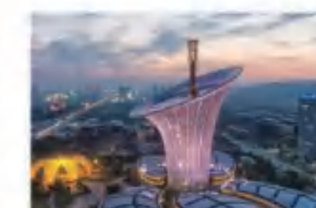
Wuhan 5497 smart apartments
